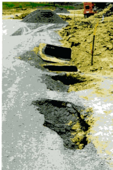
Collapsed sections of road formation following fire in HDPE pipeline
